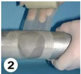
Apply the Pipe Wrap bandage around the damaged area, extending up to 50mm (2") either side of the leak to ensure complete coverage. It is important that the bandage is applied quickly as curing begins once it is taken out of the water.
